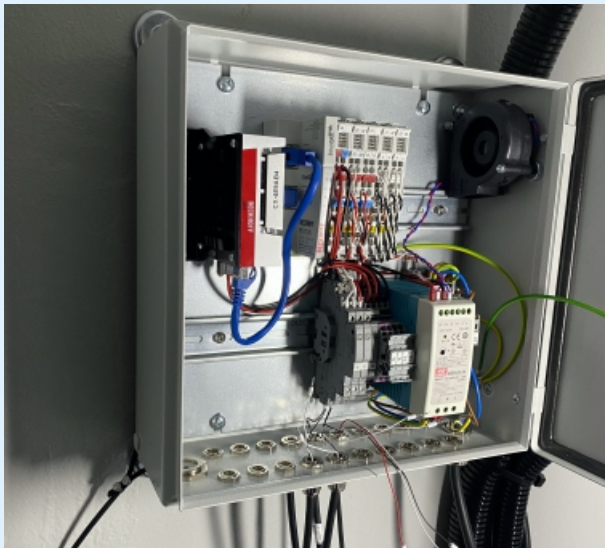
4-kanaliger Peakalyzer während der Installation in einer Windenergieanlage – 4-channel Peakalyzer during installation in a wind turbine
